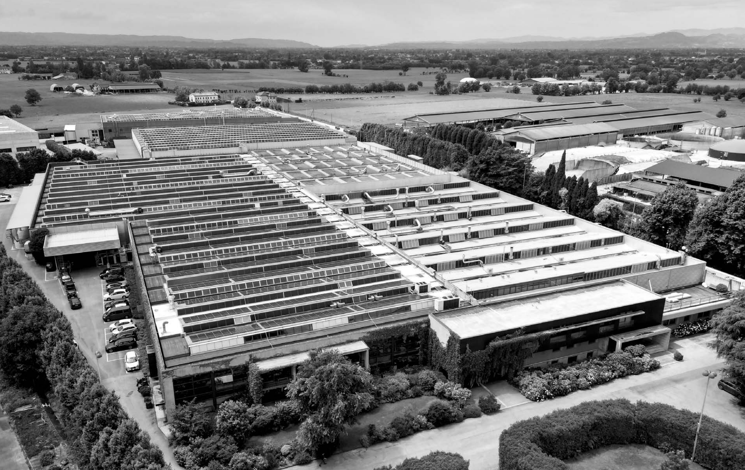
Solar panels on the roof of the Pozzoleone HQ, Italy—source: company archive
